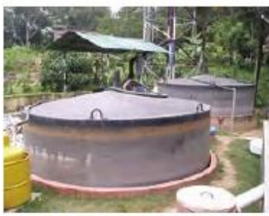
Picture 10: Floating-drum digester for market waste in India (photo: Sandecl).
