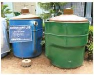
Picture 11: Above ground floating-drum digester for households in India, made of fibreglass reinforced plastic (photo: Sandecl).
