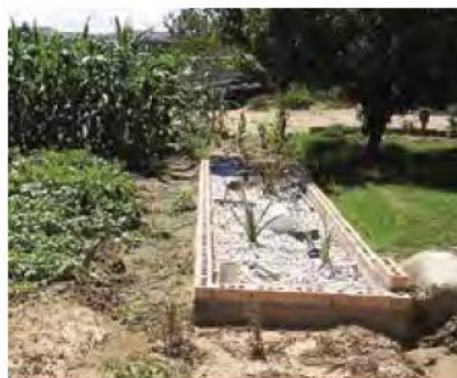
Picture 35: Newly constructed planted gravel
