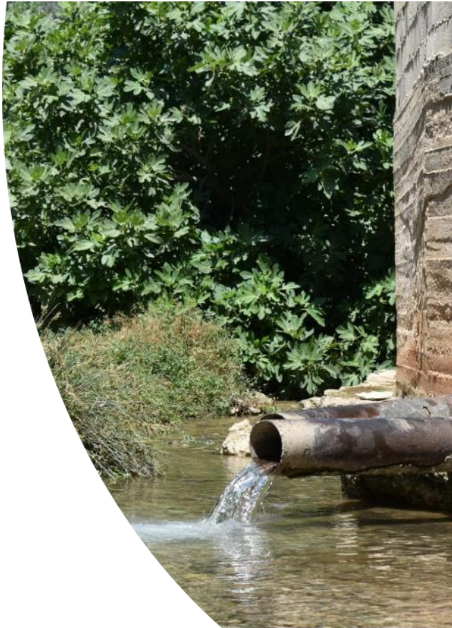
Figure 3 al-Tanoor spring is the water source for the municipal network
