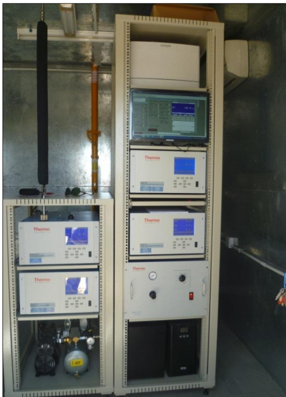
Figure (1.2) Station from inside
