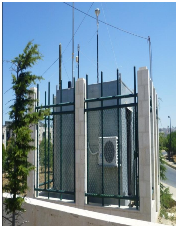
Figure (1.3) Station from outside
