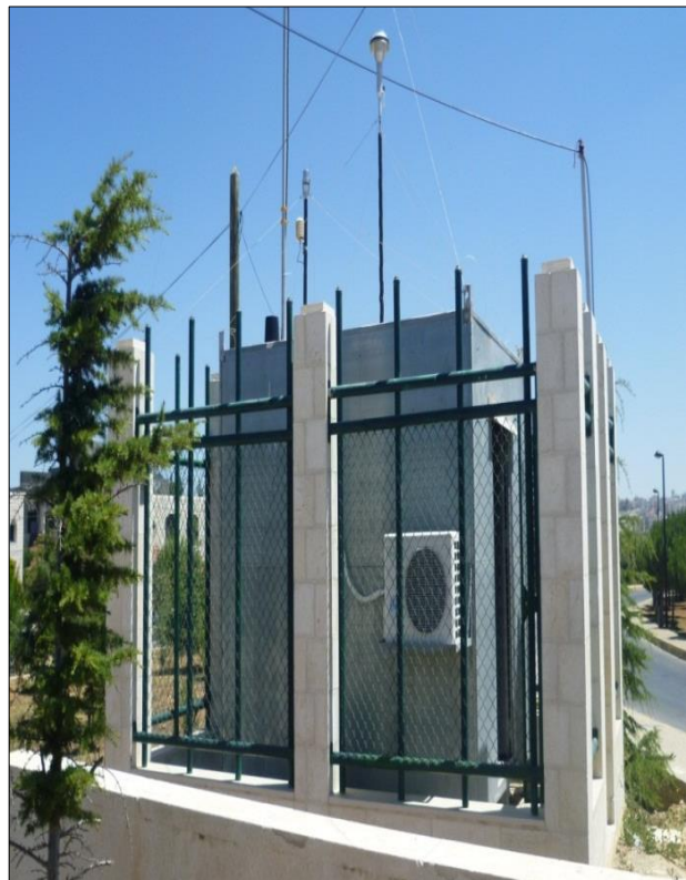
Figure (1.3) Station from outside
