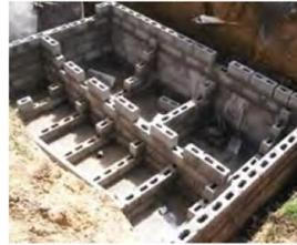
Picture 34: Anaerobic baffled reactor under
