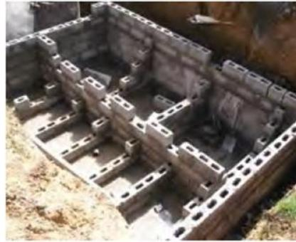
Picture 34: Anaerobic baffled reactor under
